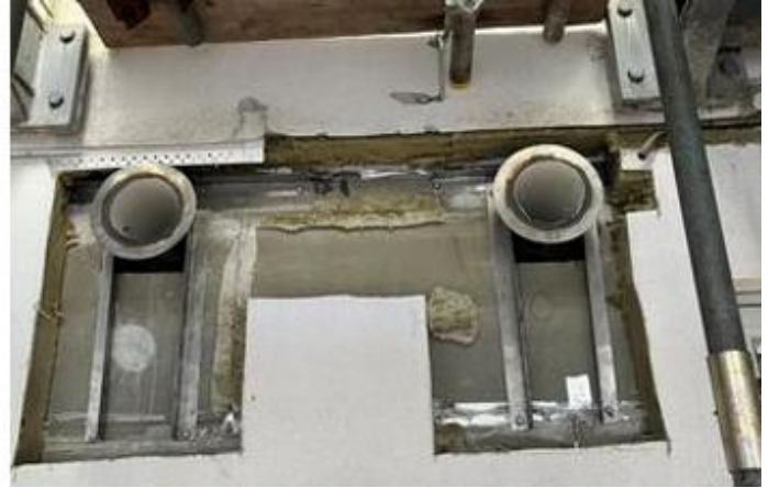
A photo showing Phase 2 North Elevation – Stainless steel sleeves installation works to EWI areas progressing
