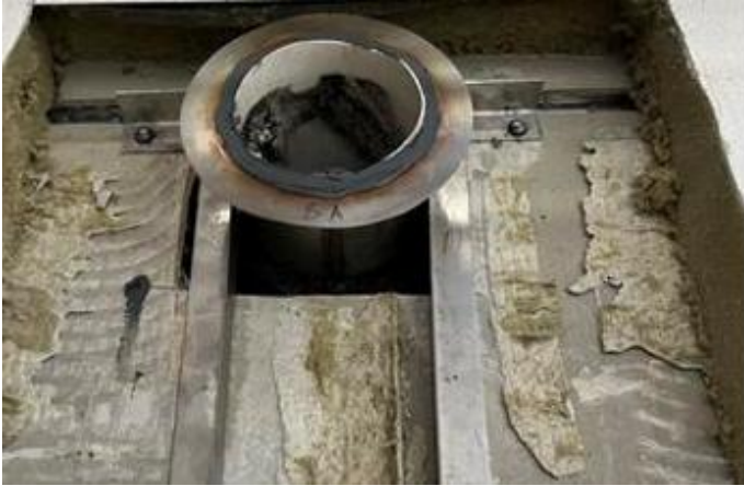
A photo showing Phase 2 North Elevation – Stainless steel sleeves installation works to EWI areas progressing
