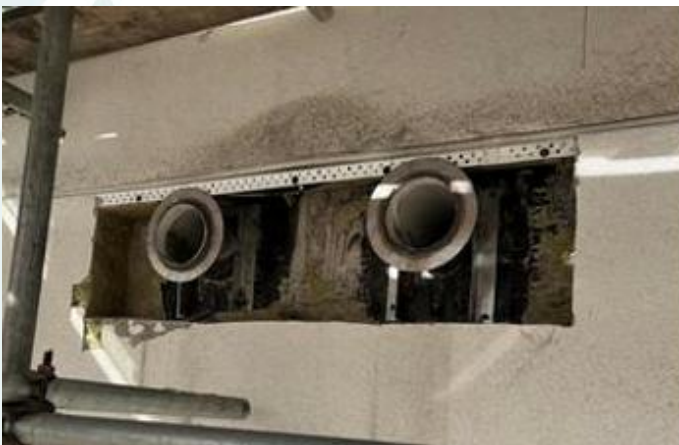
A photo showing Phase 1 South Elevation – Stainless steel sleeves installation works to EWI areas progressing
