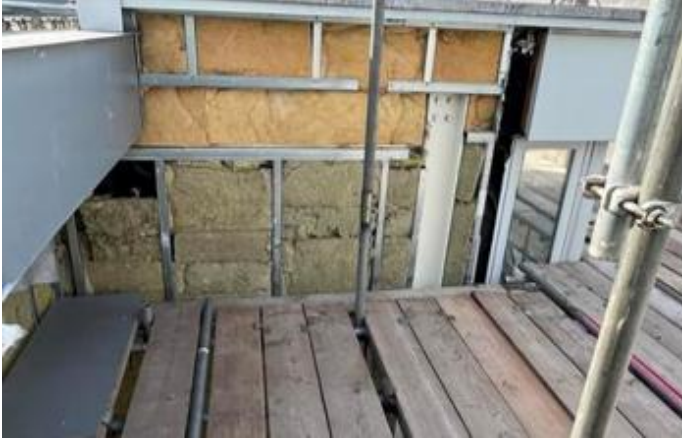
A photo showing Phase 2 North Elevation – Existing CP boards removed and steel beams exposed
